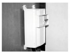
Fig. 3: Ground fault circuit interrupter (GFCI)
