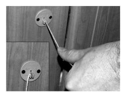
Fig. 73: String-operated baffle
