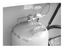
Fig. 68: Gas bottle with low pressure regulator and low pressure hose
