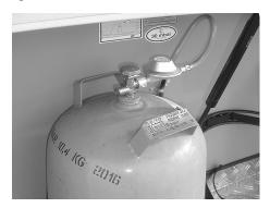
Fig. 86: Gas bottle with pressure reducing valve
