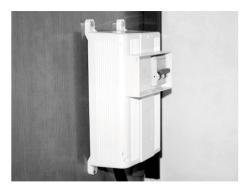
Fig. 57: Ground fault circuit interrupter (GFCI)
