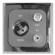
If a TV wall mounting is fitted, a 12 V socket will also be installed for powering the TV from alternate voltages.
