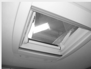
Abb. 36: Dachhaube 400x400 mm VisionStar 700x500 mm
